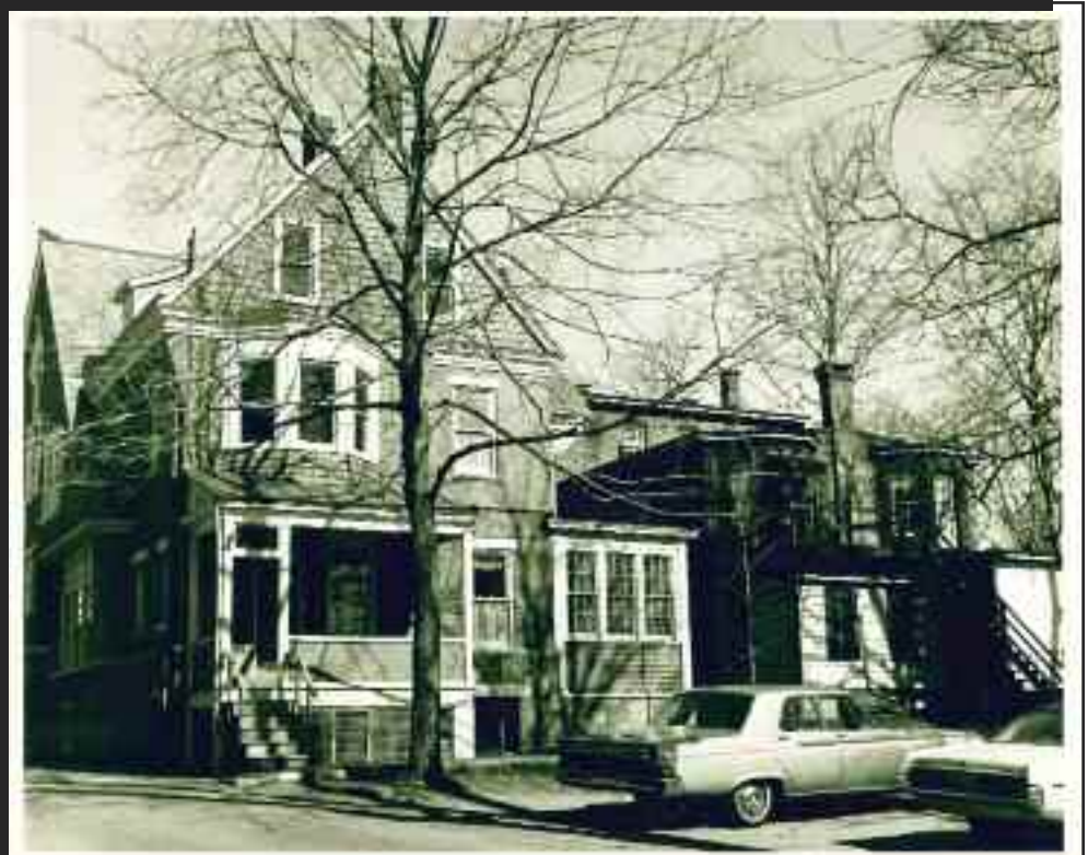
489 West State Street, Trenton Front view (L); back view (above)
